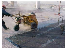
Typical application of the felts on a BUR system. Notice that throughout the system there will be felts layed in a multi-ply configuration, which provides built in redundancy. The lower roof is a two ply system installed over a nailed base sheet. Most two ply systems have a modified cap sheet installed as the top surfacing.
