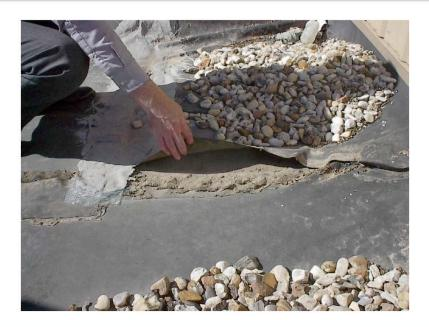
An example of an eight year old EPDM membrane shrinking. This is caused from premature aging due to damage caused from UV and heat. Most EPDM membranes are black, which absorbs heat that helps accelerate the aging process.
