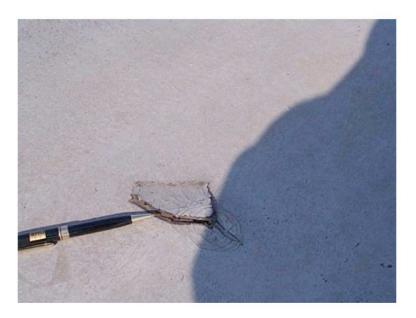
With single ply membranes only being 39-60 mils thick, they can be punctured easily. This is an example of a split that could have been caused by dropping a tool onto the membrane.
