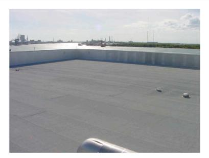
On top of the inter-ply felts, a modified cap sheet is installed. This sheet will be surfaced with either gravel or a liquid applied coating. This reinforced sheet provides added strength and protection to the system.
