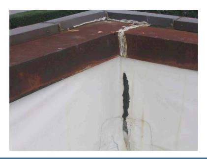
An example of a seam failure on a CSPE membrane. This seam failure allows for direct water entrance into the roofing system and the building.
