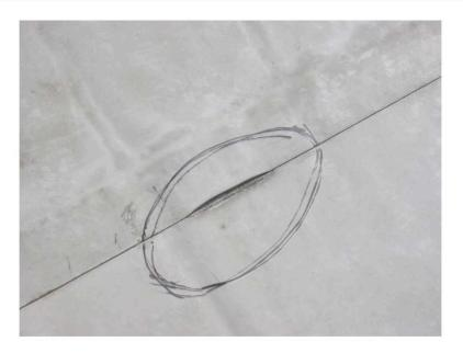
A seam failure on a TPO roof. These seams are contractor sensitive and there is only on ply of protection. the seaming of the sheet is vital to the waterproofing capabilities of the system. This is an example of poor workmanship that may or may not be caught during the final inspection.
