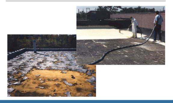
Upper Right -The application of the two part SPF is delivered to the roof in heated lines. Temperature, moisture and humidity will effect the ratios of the two materials. A trained and experienced foam crew is required for proper installation.
