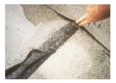
Some problems that can occur if the system is not properly installed. Here is a lap that is not adhered, typically due to an inadequate amount of bitumen being applied. Many manufacturers offer jobsite inspectors which can significantly reduce application errors such as this. This problem can easily be corrected with the use standard repair materials.
