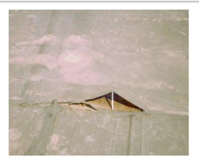
Seam failure on a seven year old EPDM roof caused prematurely from the membrane shrinking. The black surface on EPDM membranes absorb heat and UV which cause the membrane to age prematurely and shrink. AS EPDM ages, it is very difficult to permanently repair.
