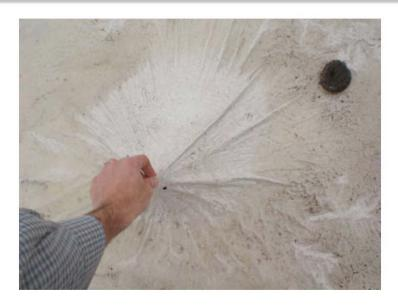
Here is a typical problem on single ply roofs. Notice the tent like profile of the sheet. This is the result of fasteners backing out through the membrane causing punctures were water can enter the building.
