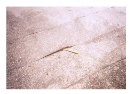
Another example of a problem that can occur if the system is not properly installed. Here is a lap that is not adhered, typically due to an inadequate amount of bitumen being applied. Many manufacturers offer jobsite inspectors which can significantly reduce application errors such as this. This problem can easily be corrected with the use standard repair materials.
