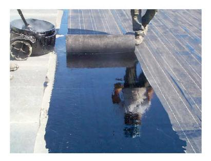
Application of the felts. Notice the overlapping of the sheets to ensure that there is more than one layer of protection trough out the system.
