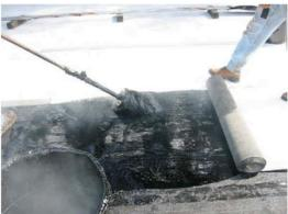
A typical application of the felts that will be beneath the modified cap sheet. The lapping of the felts results in multi-ply redundancy being built into the system.
